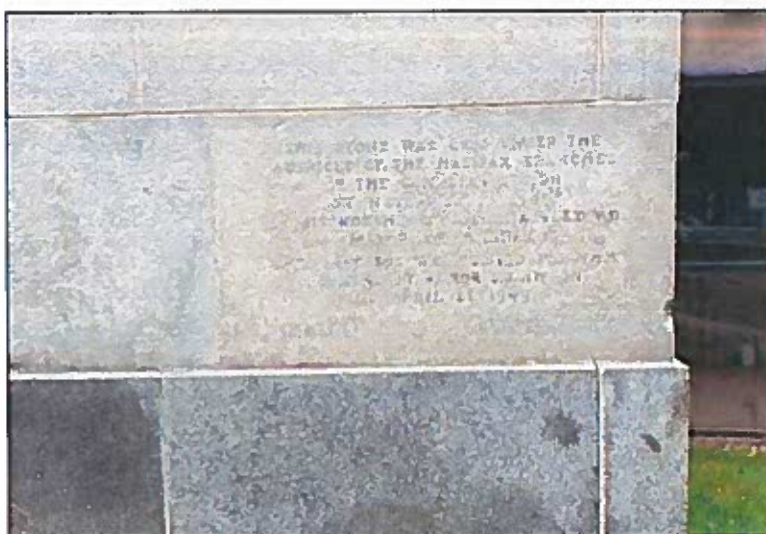
Plate 7: Cornerstone of the former Halifax Memorial Library.
