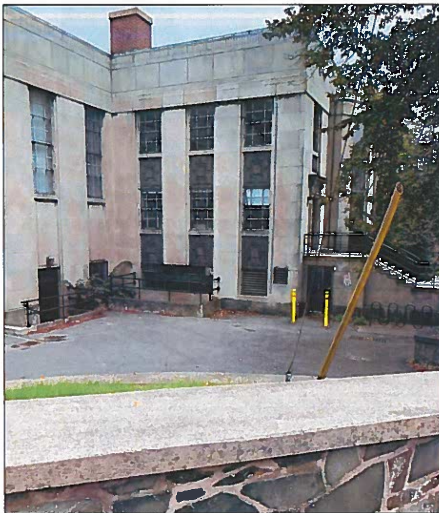
Plate 15: Rear of Former Memorial Library Building from sidewalk on Brunswick Street. Note storm drain on right by bicycle racks. Facing southeast. September 28, 2020.
